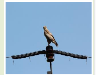
Installation of bird protection devices
